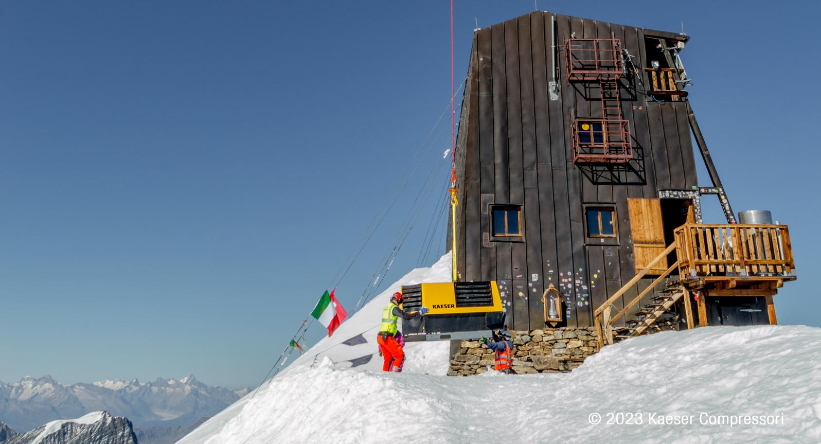
**In a challenging Alpine setting at 4,554 meters, the Regina Margherita refuge undergoes a stability project led by PoliMi University and the Italian Alpine Club. Using Mobilair Kaeser compressors, the team successfully drills and installs sensors to monitor permafrost conditions and rock stability.**
